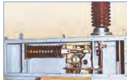
Spring Mechanism 145kV - Opening Spring (Rear View)
