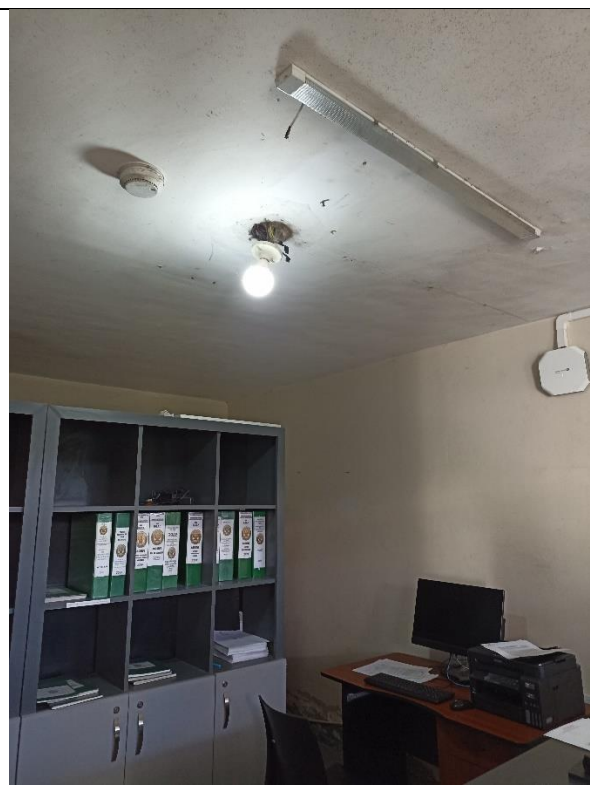
CAMBIO DE LUMINARIA LED 60x60x48W
