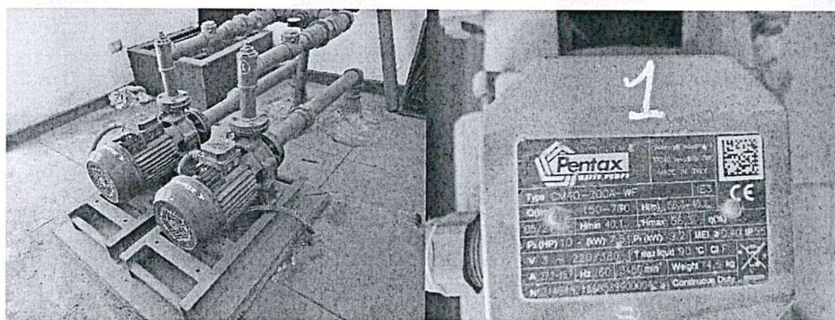
Electrobombas de 10HP, 220V, Trifásico, 60Hz (02 Und)
