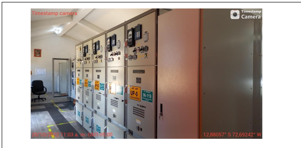
Figura 47: Celdas de Media tension, SE Urpipata
