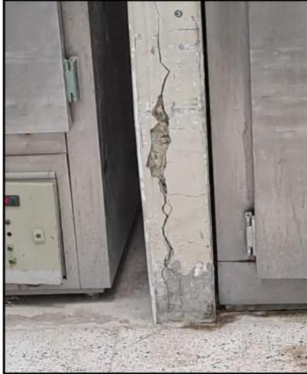
IMAGEN 11: FISURA EN MURO, EN SALA DE MORTUORIO
