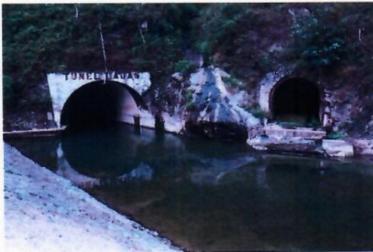
Photo N°08 and 09: lajas tunnel that captures water from the lajas stream and exit tunnel.
