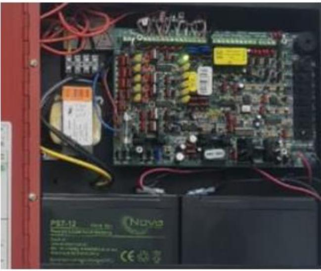
The interior of a fire alarm control panel is shown, revealing a complex circuit board with various electronic components, including resistors, capacitors, and integrated circuits. Several colored wires (red, blue, yellow) are connected to the board. Below the board, two black batteries are visible, with the 'Novus' brand name and '12V' rating partially visible. |
