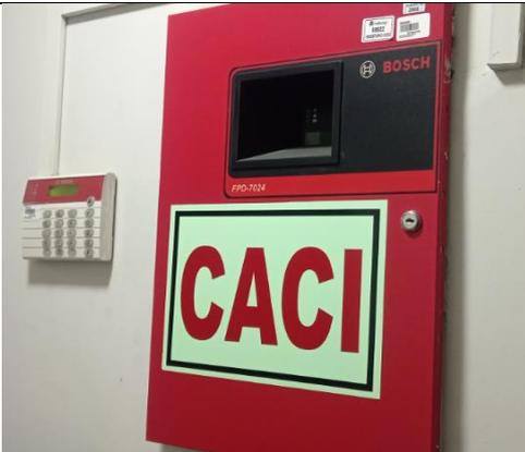
A red fire alarm control panel is mounted on a white wall. It features a small digital display and a keypad. A prominent white sign with the letters 'CACI' in red is attached to the front. The Bosch logo is visible at the top right of the panel.                                                                                                                         |
