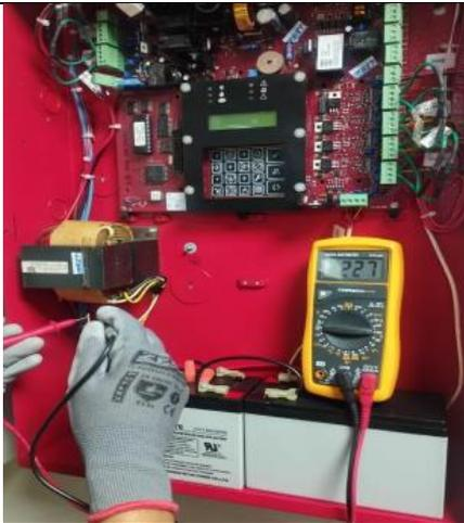
A close-up photograph of a fire alarm control panel. A person wearing a grey work glove is using a yellow digital multimeter to test the circuitry. The panel is red and has various wires and components visible.                                                                                                                                    |
