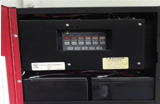
A photograph of a fire alarm control panel mounted in a red cabinet. The panel is black and features a keypad with several buttons and a small display screen. Two large black batteries are visible at the bottom of the panel. A yellow label is attached to the panel.                                                                           |
