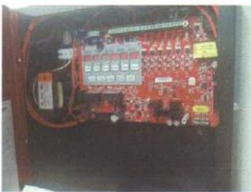
The interior of a fire alarm control panel is shown, focusing on the main circuit board. The board is populated with numerous electronic components, including resistors and integrated circuits. Wires are connected to the board, and the overall layout is organized for functionality.                                                                                  |
