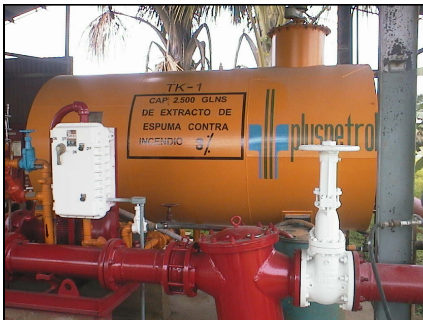
Figure 29. Corrientes Fixed Foam Tank and Proportioning System
