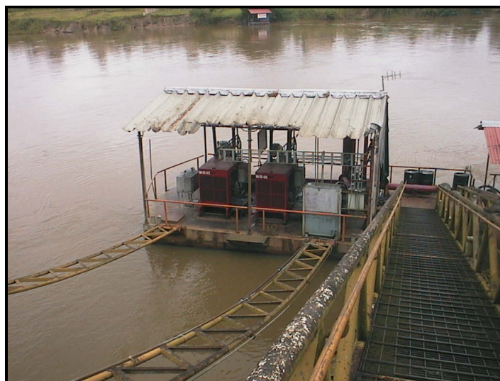
Figure 25. Corrientes Battery 1 and 2 Fire Pumps
