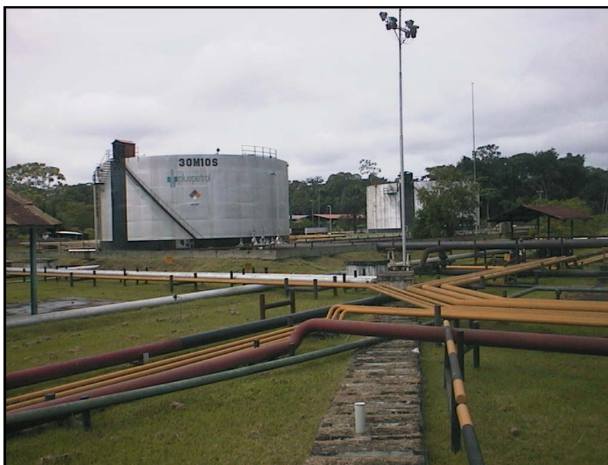
Figure 30. Fixed Foam Lines (yellow) Feeding Crude Oil Storage Tanks at Corrientes Battery 2
