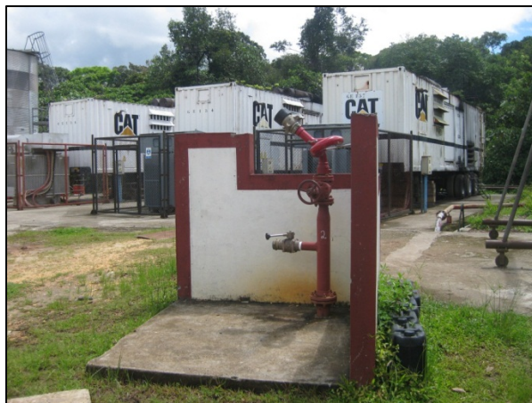
Figure 26. Monitor Nozzle Protection (with a radiant heat shield) at the Pavayacu Electrical Plant
